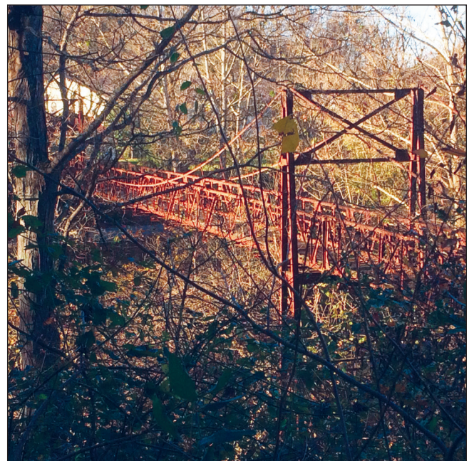
Historic bridge over Little Coal River 2017
